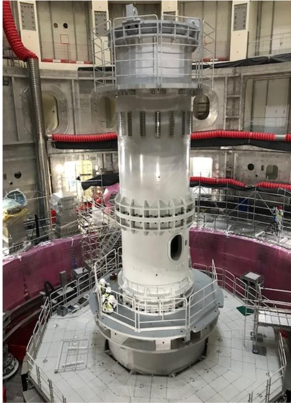
Central Column installation in the Pit
