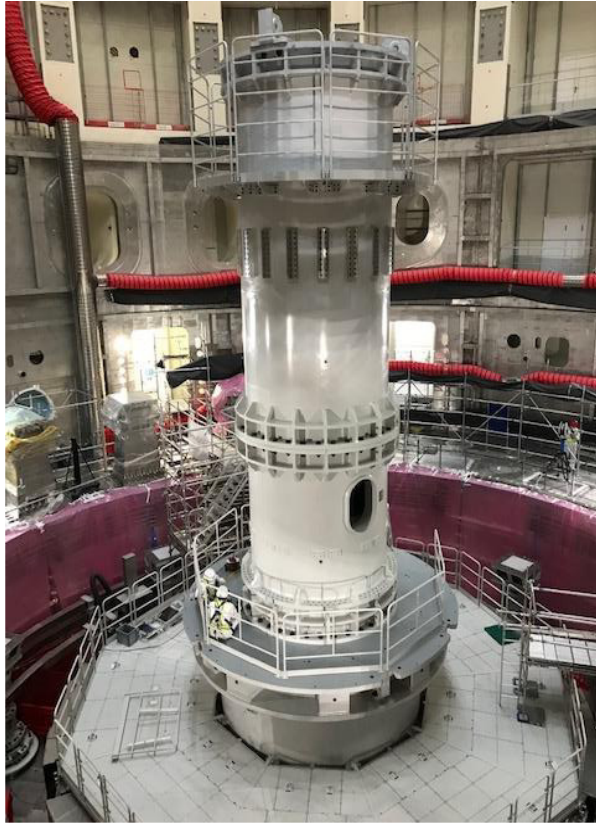
Central Column installation in the Pit
