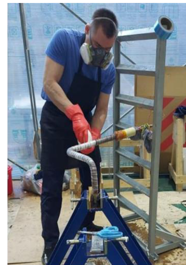
Applying glass tape
