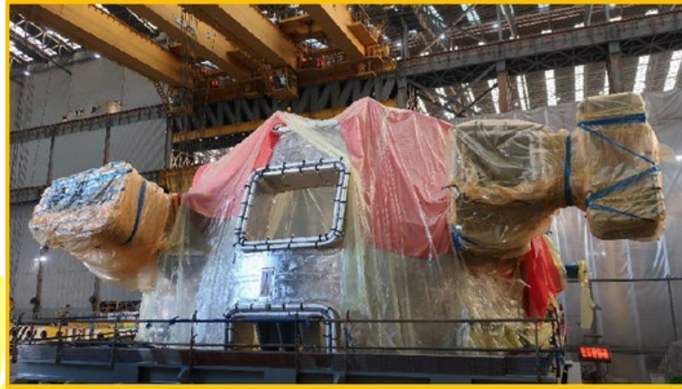
3 of 4 Vacuum Vessel sectors complete
