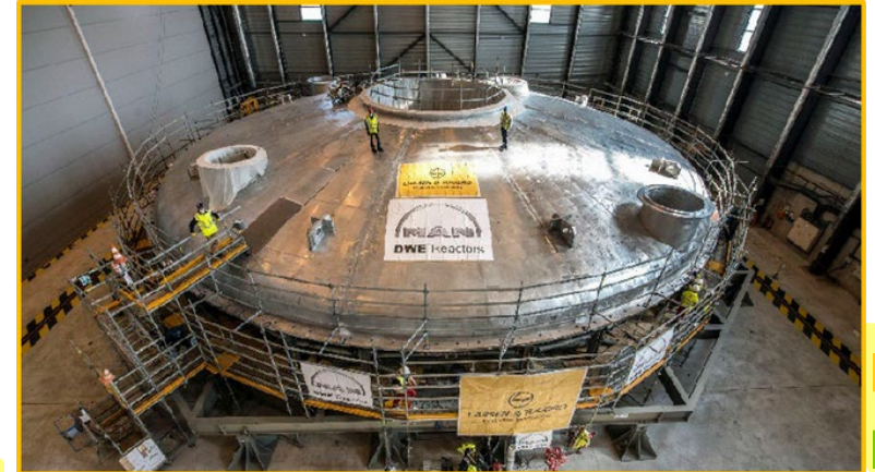
Cryostat Manufacturing is complete
